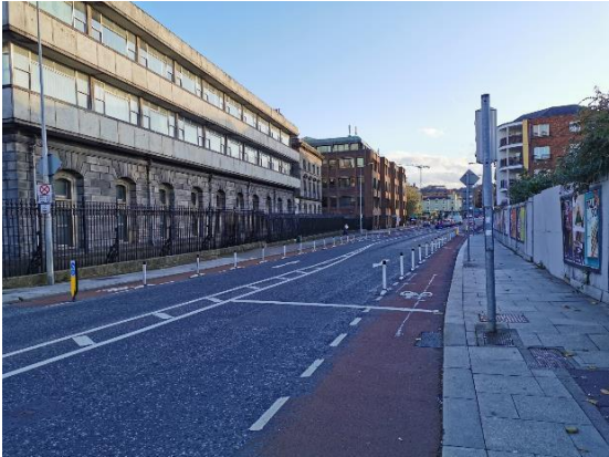
Figure 7-16 Surface treatment in existing cycle lanes
