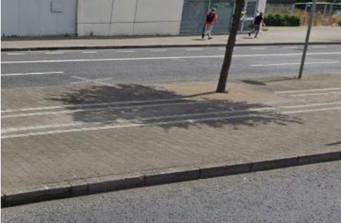
Figure 7-15 Concrete Paved Median
