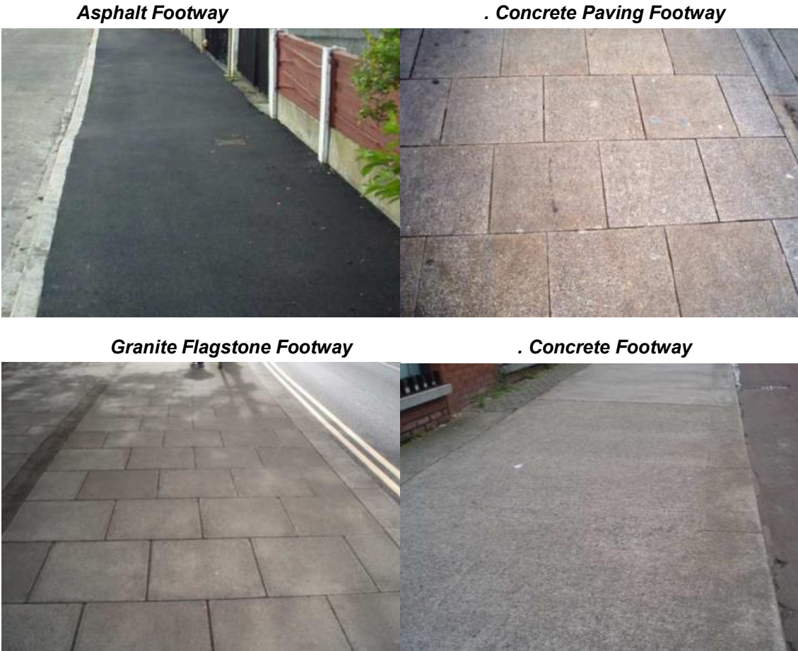
Figure 7-18: Footway Paving Types
