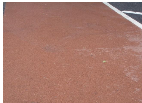
Resin Based Surface (Treatment (High Friction Surfacing Type 2))
