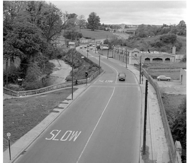
Figure 7-3 Finglas Road at River Tolka in 1971 prior to the widening to dual carriageway
